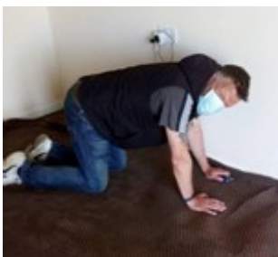
Bill Davies, Community Maker laying carpet to prepare a home to facilitate a discharge
